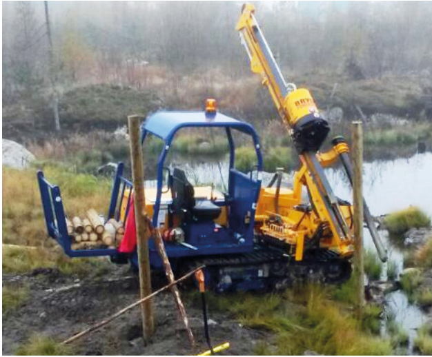
The Bryce HD180 erecting reindeer and elk fencing on the Artic Circle in Finland
