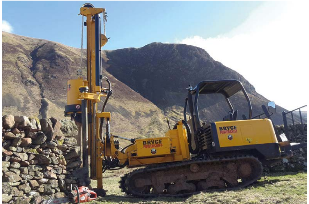
Driving straining posts in hard country up Scaur Glen
