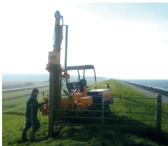
Working on a dike which is man-made. The ground is very hard. Some dikes have 26mt driven sheet metal piles for stability. Sea is on the right - 7 mts below sea level on the left.
