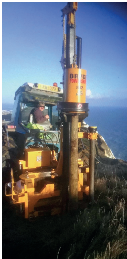
Working on chalk and flint on the White Cliffs of Dover
